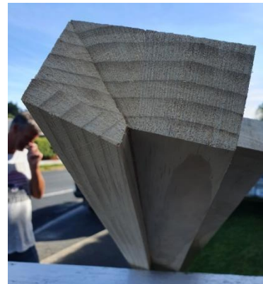
Graeme fitting and trimming the square corner detail
