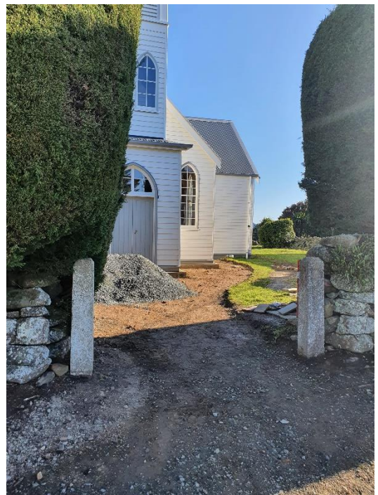
Getting ready for the new paving
