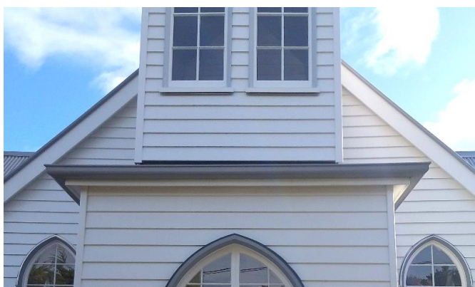
PVC guttering to Foyer now replaced
