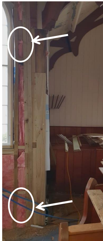
(Compare stud spacing top and bottom)
