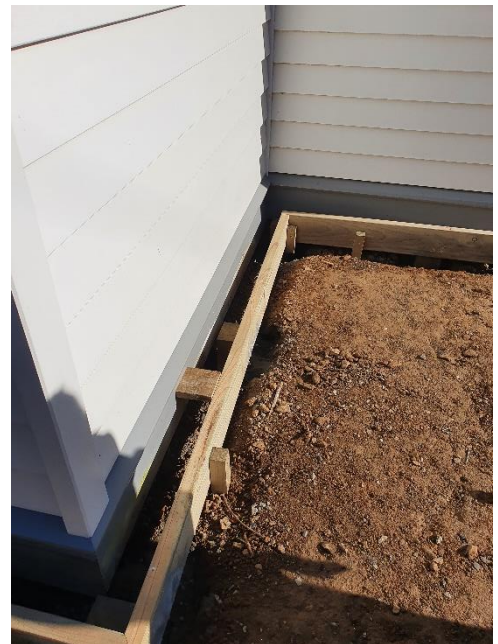
Preparing for the new strip drain around the front of the church
