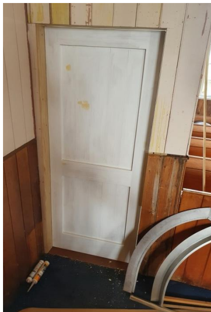
New side door installed
