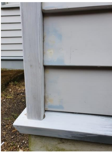
External square corner detail
