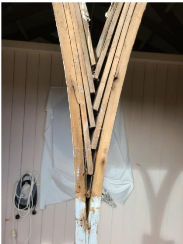
Walter Riddell's unique construction of the large NE window is revealed
