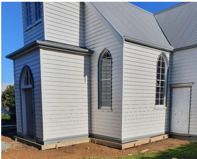
Preparing for the new strip drain around the front of the church
