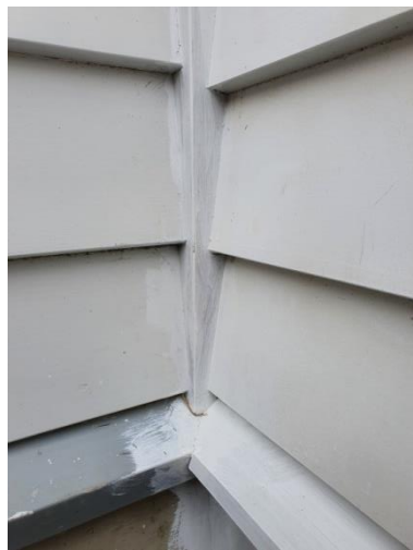
Internal square corner detail
