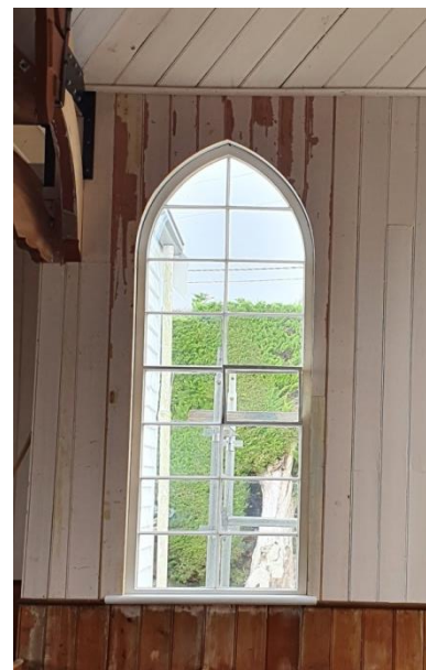
Interior lining around windows reinstated
